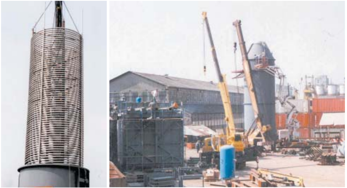
Figure 2. Mounting of the start-up heater.
