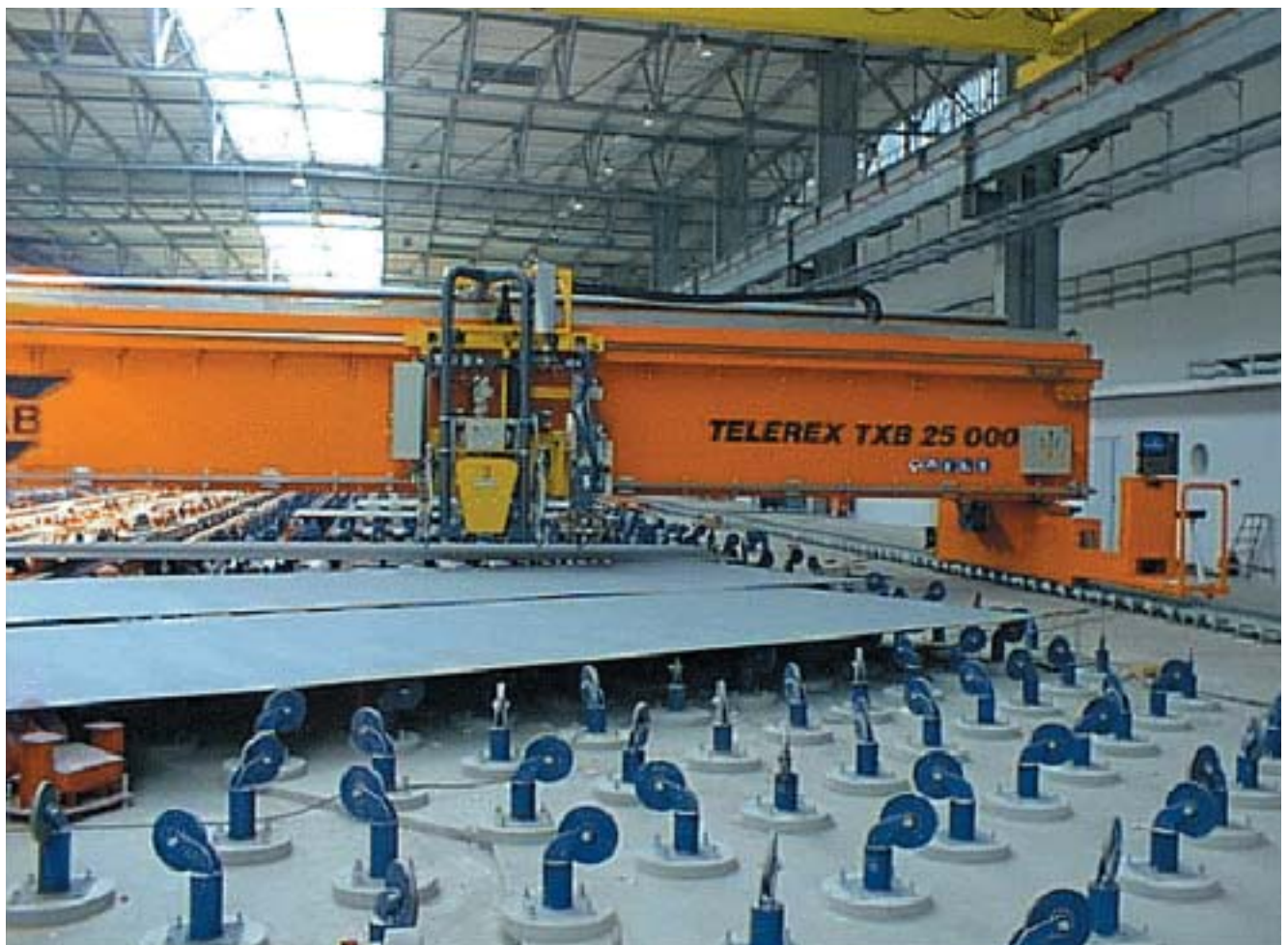
Figure 6. Grinding device installation on panel machine for a shipyard in France.
