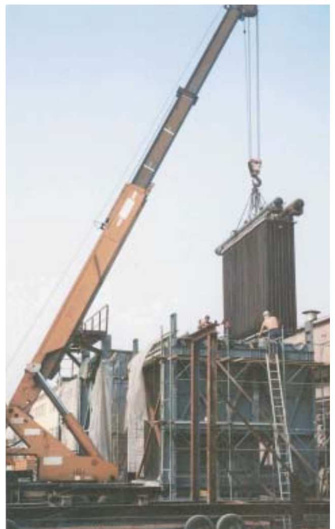
Figure 4. Mounting of waste train water heater.
