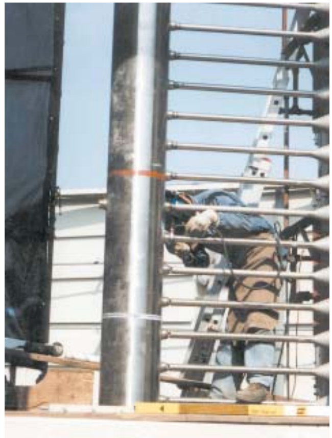
Figure 1. TIG welding of Inconel pipes.
