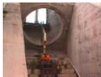
Figure 7 – Upper part of a penstock
