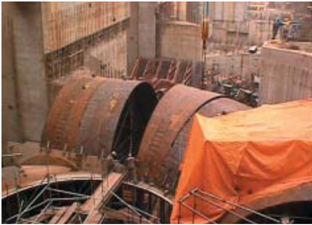
Figure 4. Details of protection tent – assembling of a spiral.
