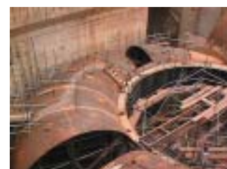
Figure 6. Assembling of a spiral
