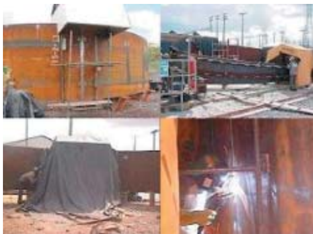
Figure 3. Details of protection tent – pre-assembly.
